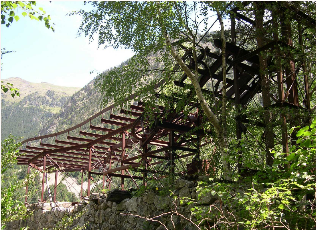
Luisa cableway arrival station
